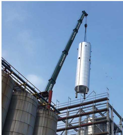
New stirring tank in the G 28 Production of oils (right)
